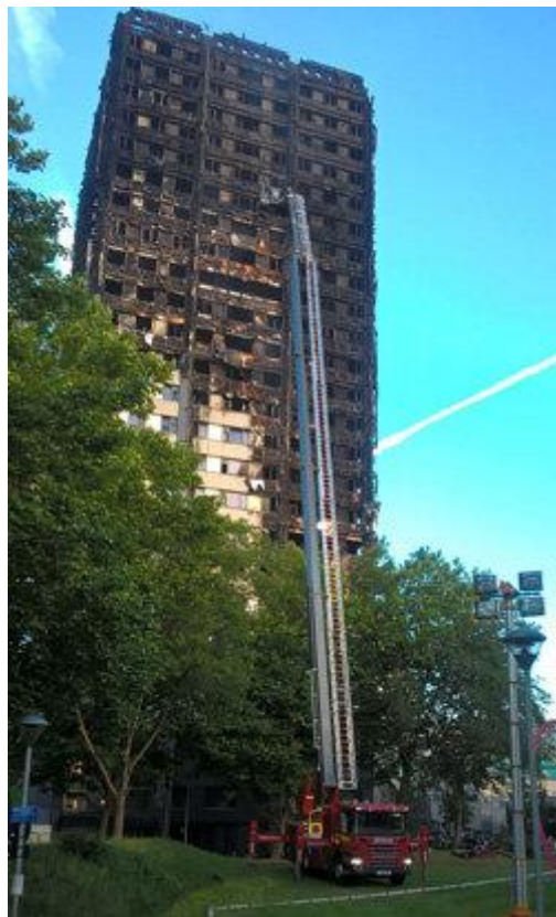
Figure 1 - Surrey Fire and Rescue Rosenbaur 43m ALP pitched on grass at Grenfell 5
